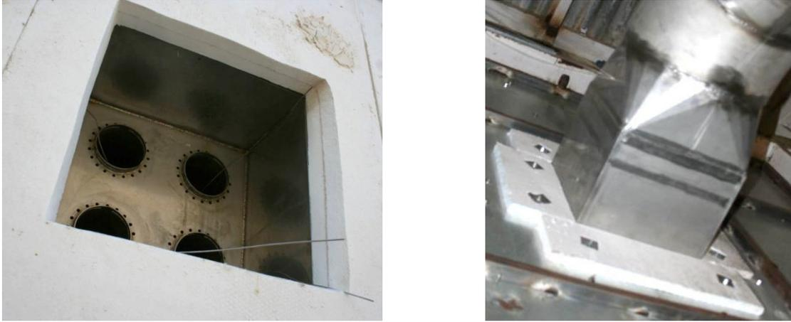
**FIGURE 5.** 2 x 2 array test loop installed at SSPS-CRS tower – front view without cups (left) – rear inside view (right)
