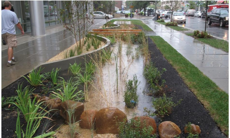
*Retention systems capture and store stormwater runoff and pass it through a filter bed of engineered soil media composed of sand, soil, and organic matter. Rain gardens are a common example of a retention system. Image credit: DOEE*
